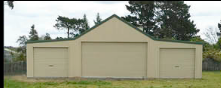
42) Aussie Barn with Three Roller Doors 6m x 9m x 3.2m with 30° roof with 3m lean-to Classic Cream™ walls | Pale Eucalypt® trim
